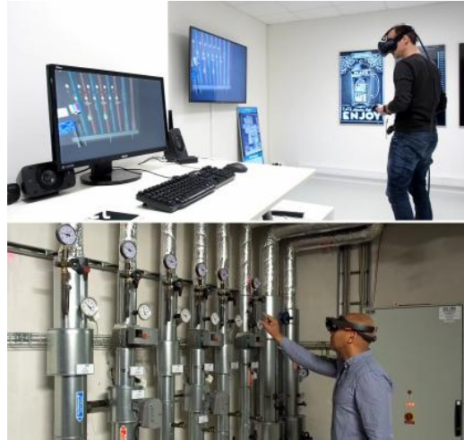
Figure 3.12: Using BIM and a shared VR(top)/AR(bottom) environment for remote support ( Image: Exozet )
