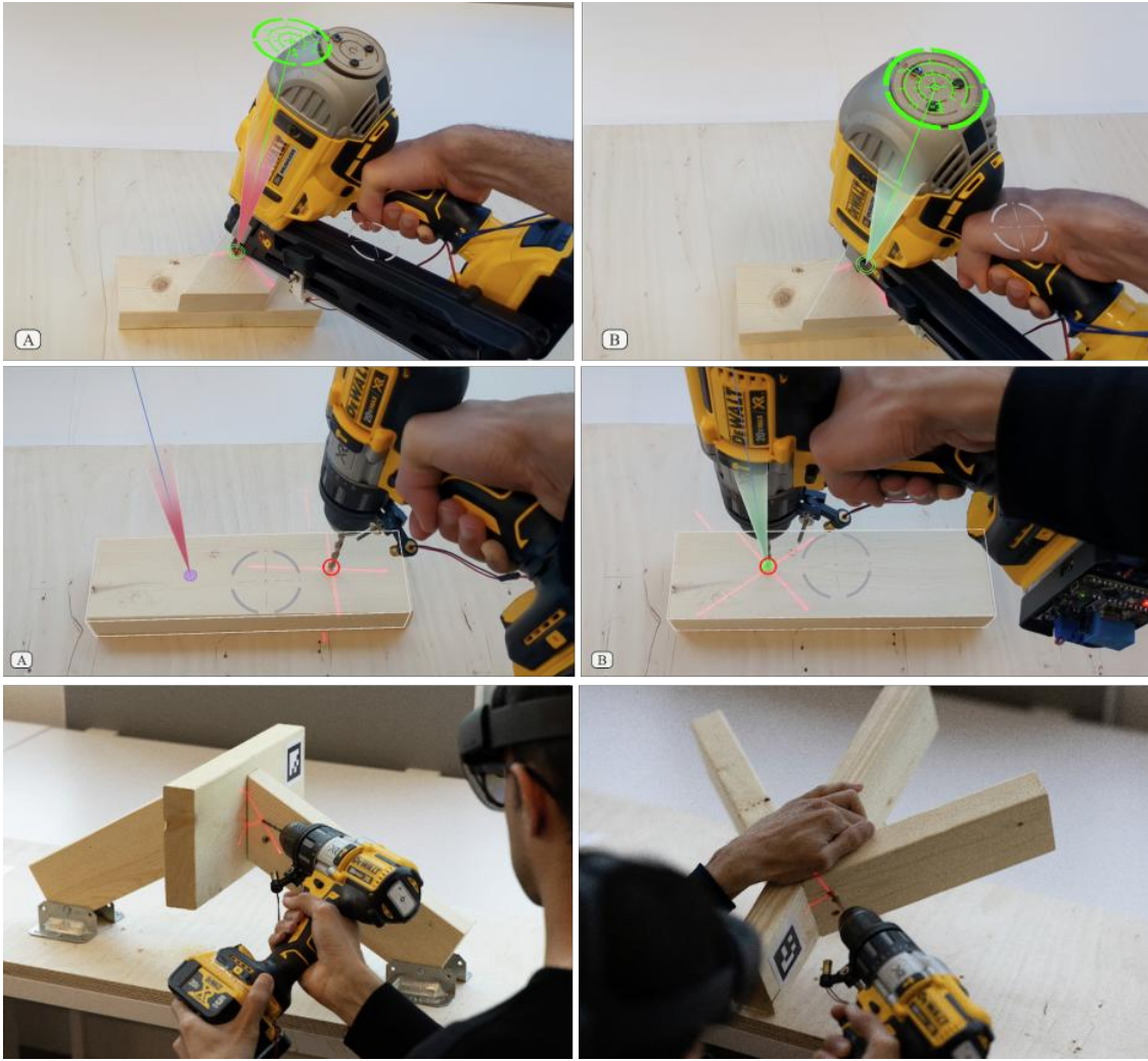
Figure 3.2: Using AR for assisting workers in timber connection execution tasks by giving visual indications of the points where the worker has to drill or apply joint screws. The system proposed by Fazel and Adel [109] can also track power tools to detect positional and orientation errors.
