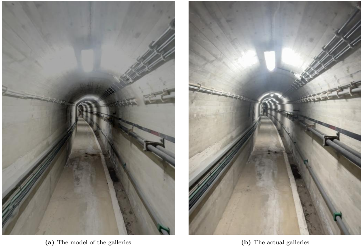
Figure 5.18: The galleries models built for GalleriesVR used a high level of visual detail, with photographic textures and high polygon count for smoother shapes, which made it possible to reproduce (a) the real galleries in the Cabril Dam (b) with high fidelity (Soares [149])
