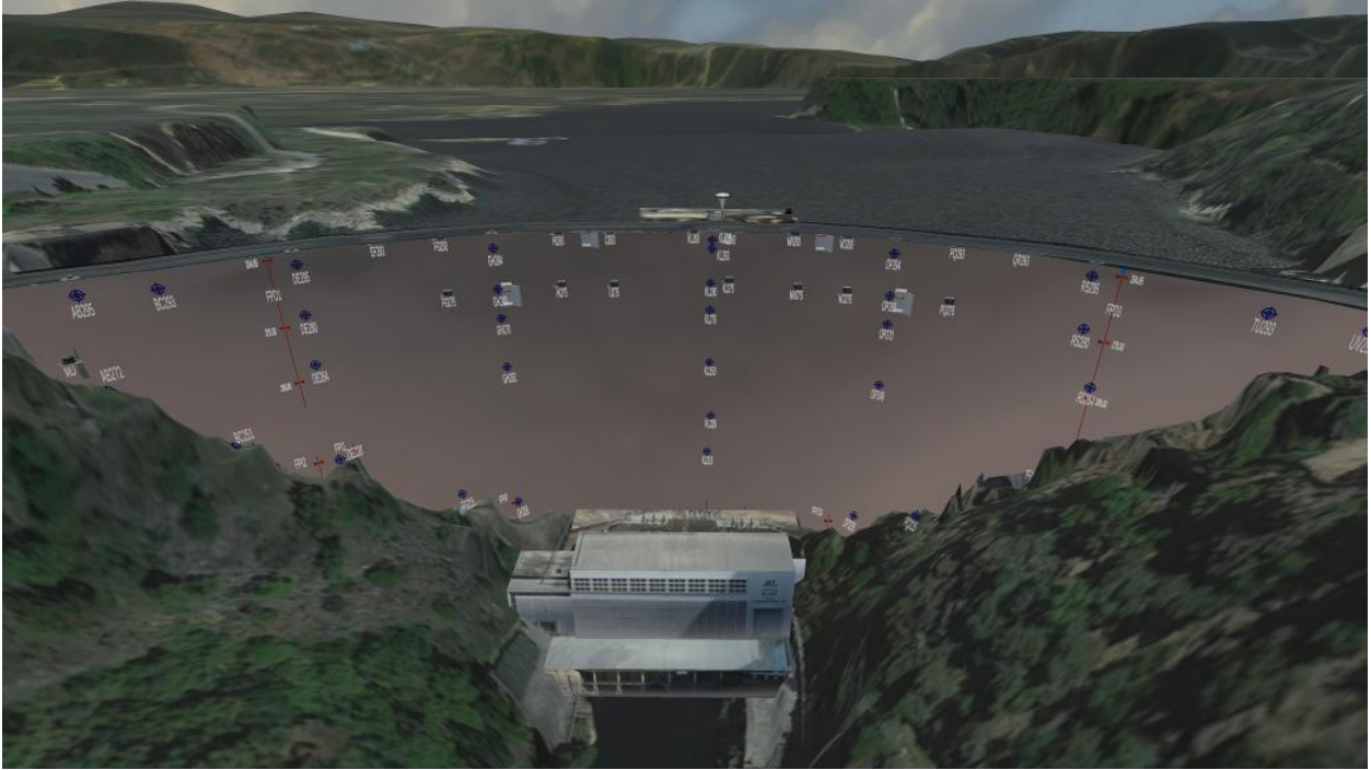
Figure 4.10: An ‘X-ray’ overview of the networks of sensors located inside the model of the Cabril Dam represented in DamVR ’s virtual environment [164].
