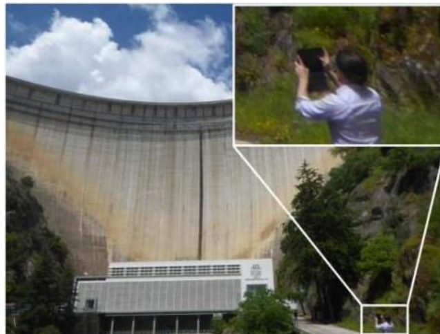
FIGURE 30.2 On-site augmented reality-enabled structural health monitoring sensor network visualization with a tablet.
